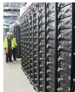
Typical Rack (Ref. 2). 6 MW Leighton Buzzard
